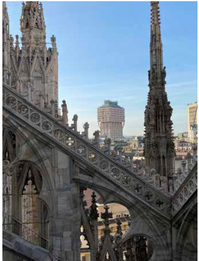
Above: From the rooftop of the Cathedral (which we will visit) there is a stunning panorama over Milan, where the abundance of twentieth century architecture will be revealed. The tower in the center is the Torre Velasca, by Belgiojso, Peressutti, and Rogers of 1958.
