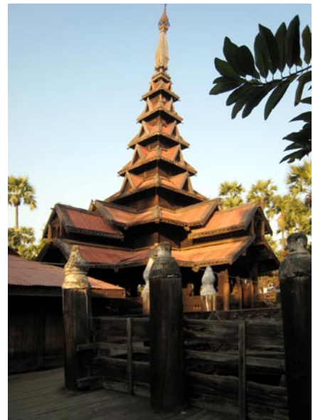
Bagaya Kyaung (Monastery), Inwa, near Mandalay, Built entirely of teak in 1834.
