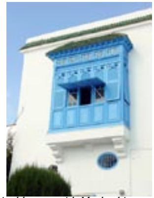
One of the typical houses with Mashrabiya window, Sidi Bou Said
